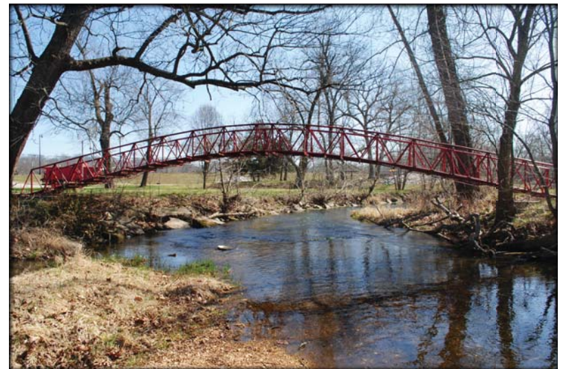
FIG. 2.44 Bridge at Crane Park
