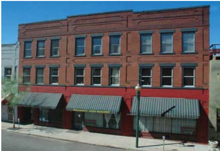
FIG. 4.21 Downtown Multi-use building
