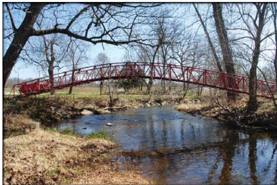
FIG. 2.48 Bridge at Crane City Park
