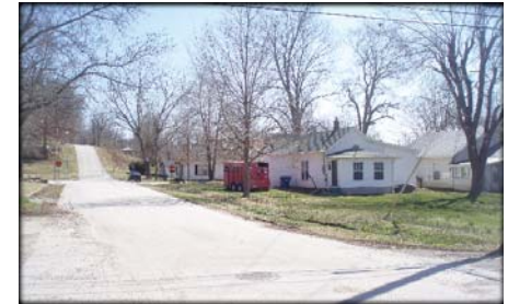
Fig. 2.11 Typical Residential Road
