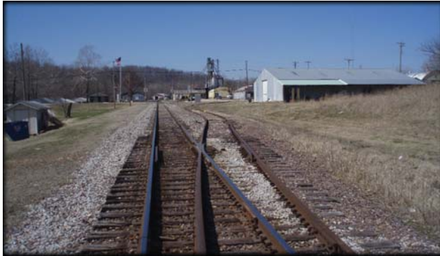
FIG. 2.27 Rail through Crane
