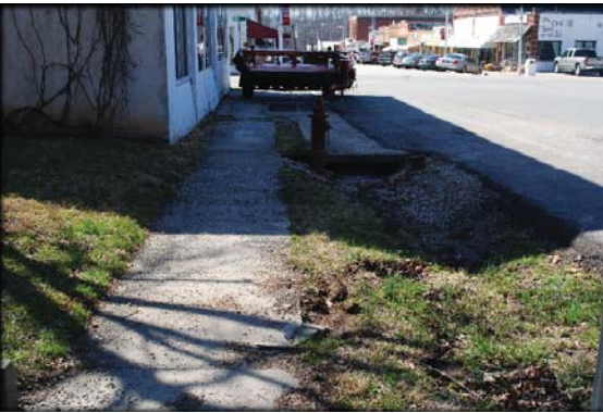
FIG. 2.29 Sidewalk in Crane
