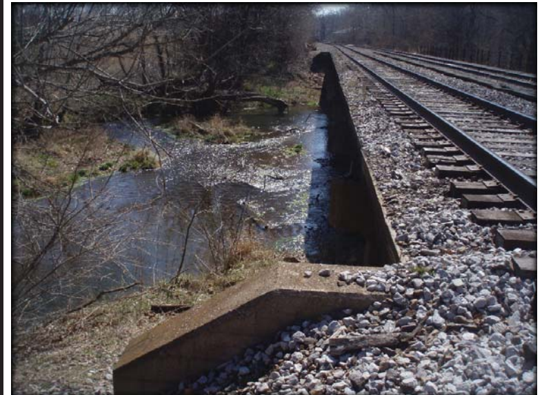
FIG. 2.54 Railroad crossing Crane Creek
