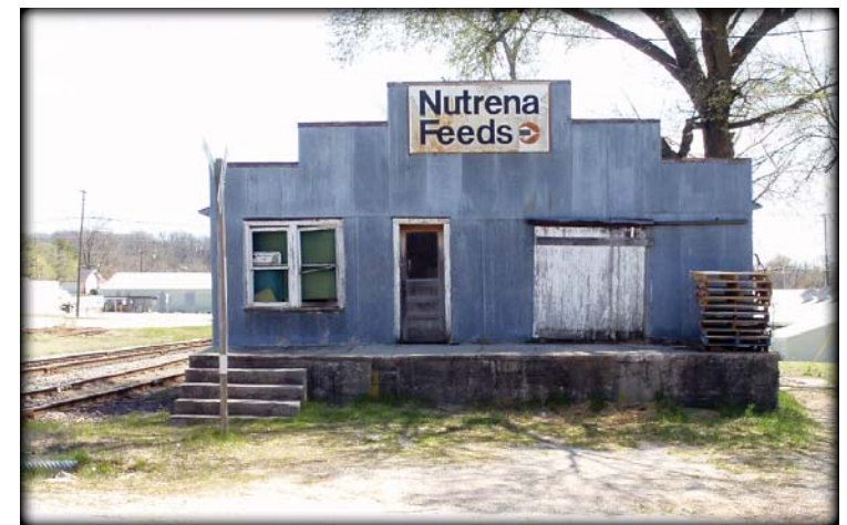
FIG. 2.41 Empty Feed Store
